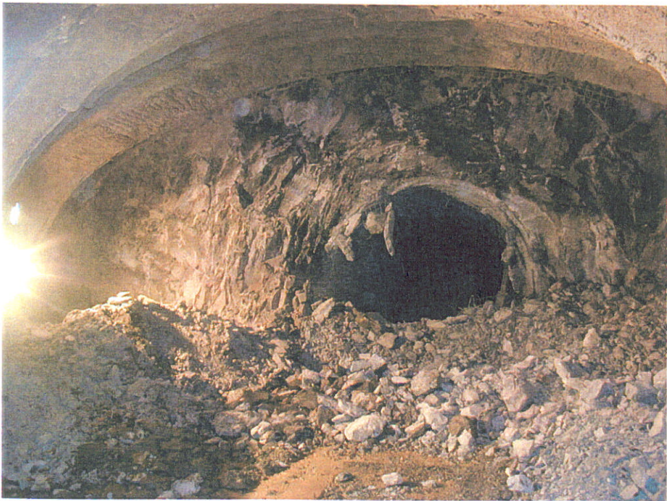
Figure 9 – Face of the enlargement section
