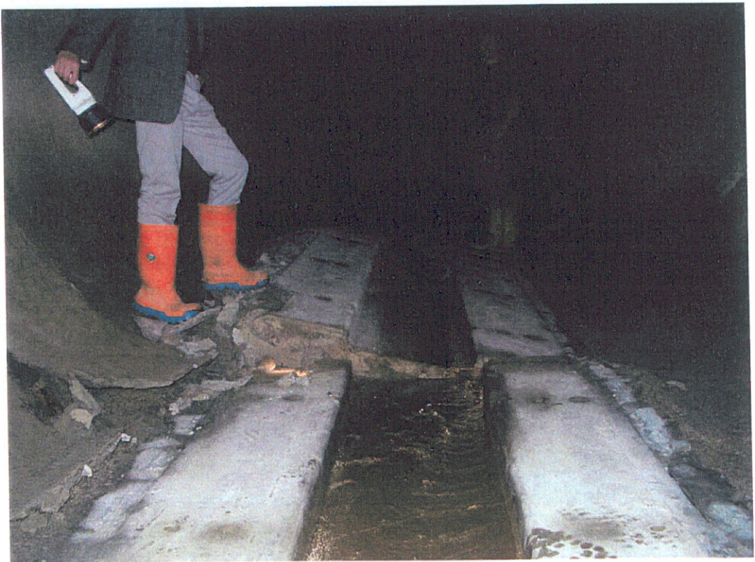
Figure 5 – Variation of the invert heaves from one segment to the next
